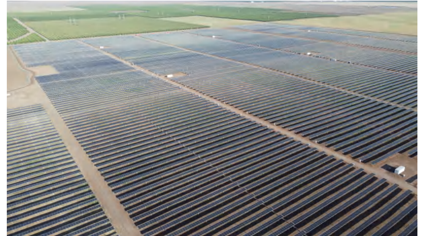
• 73 MWp Tulare County, California, USA
